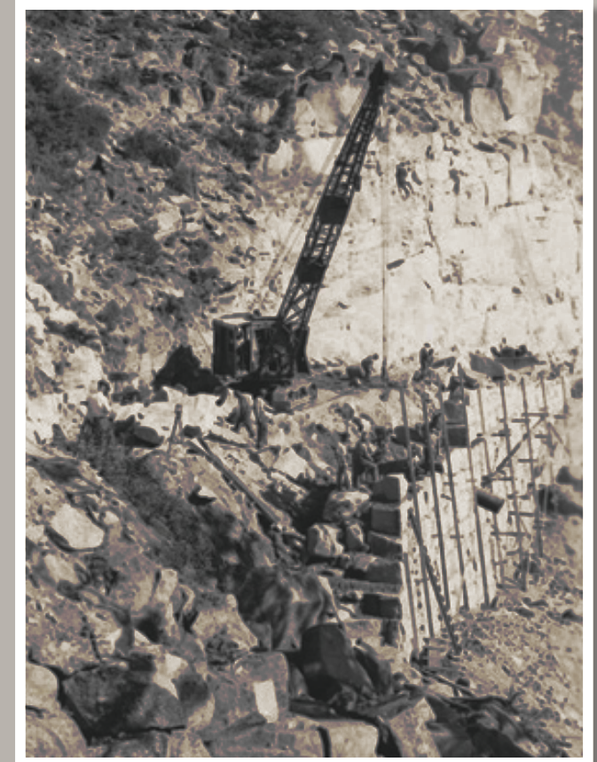
Construction of retaining wall, c. 1937 (Caltrans Transportation Library)
