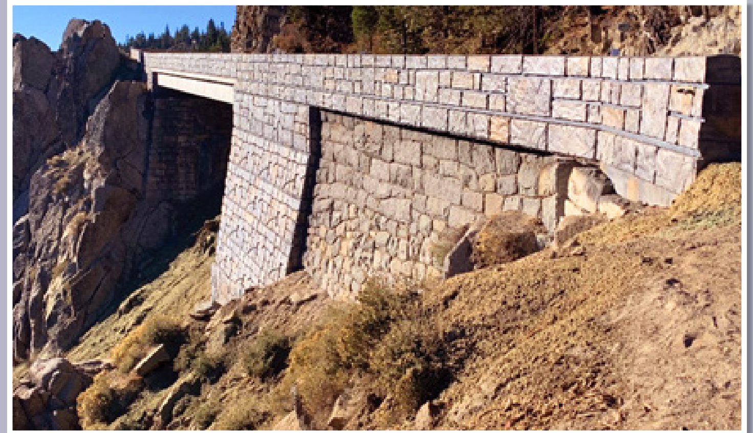
New Echo Sidehill Viaduct (Caltrans District 3 files)
