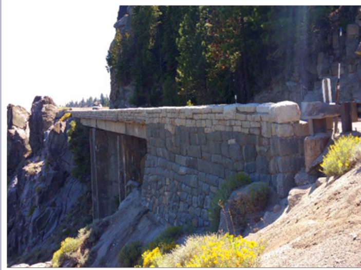
Echo Summit Sidehill Viaduct before replacement (Caltrans District 3 files)
