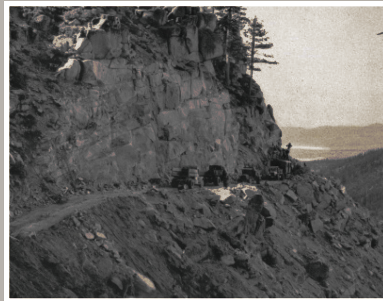
"On sheer eastern cliffs of Echo Summit power shovel is making final cut for Meyers grade relocation. Lake Tahoe in distance" (CHPW, August 1938:5)
