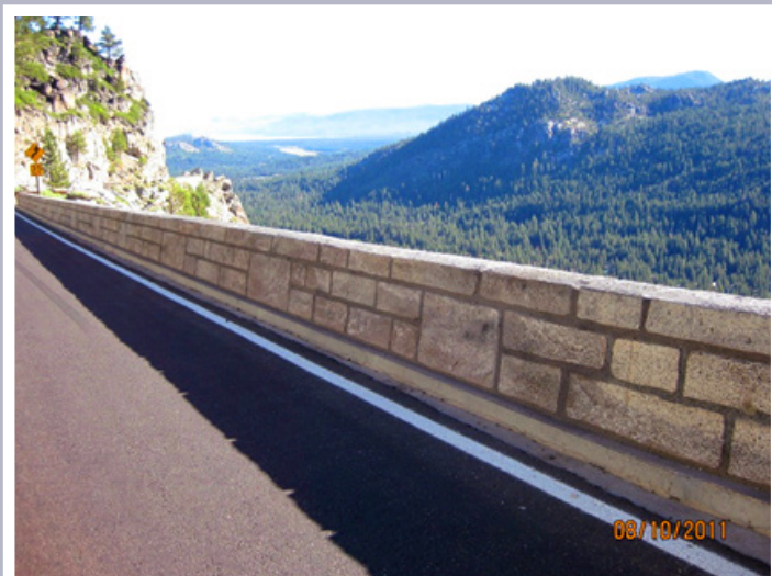
Modified concrete barrier at Echo Summit (Caltrans 2011)
