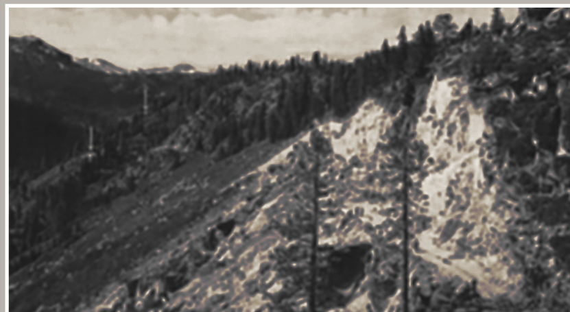
"View of new construction on Echo Summit looking south toward Luther Pass. Arrows indicate portions of old Hawley Grade" (CHPW, August 1938:6)
