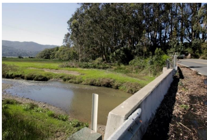
Figure 2. Culverted Creek at Millerton
