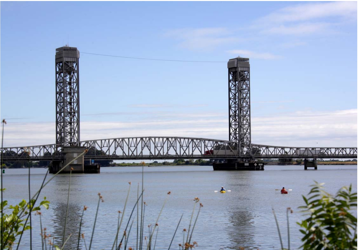
Rio Vista Bridge across the Sacramento River and shipping channel.
