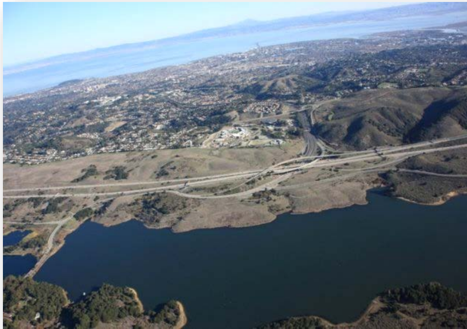
Crystal Springs Reservoir at I-280 and SR 92
