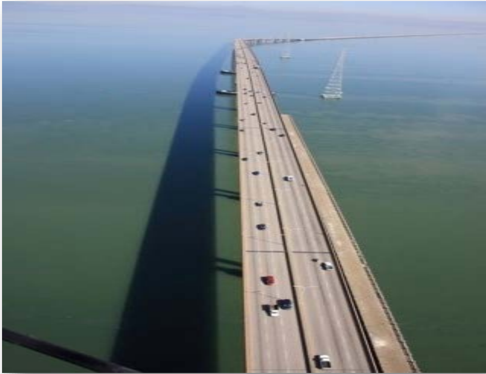
Aerial San Mateo-Hayward Bridge looking east
