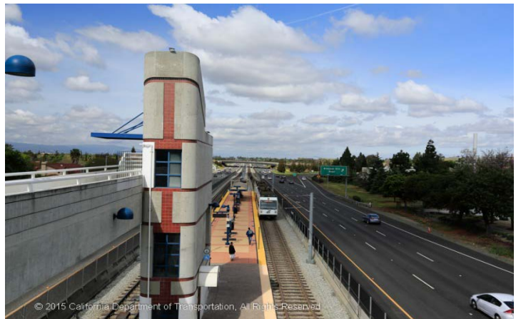
VTA Light Rail Station at Cottle Road
