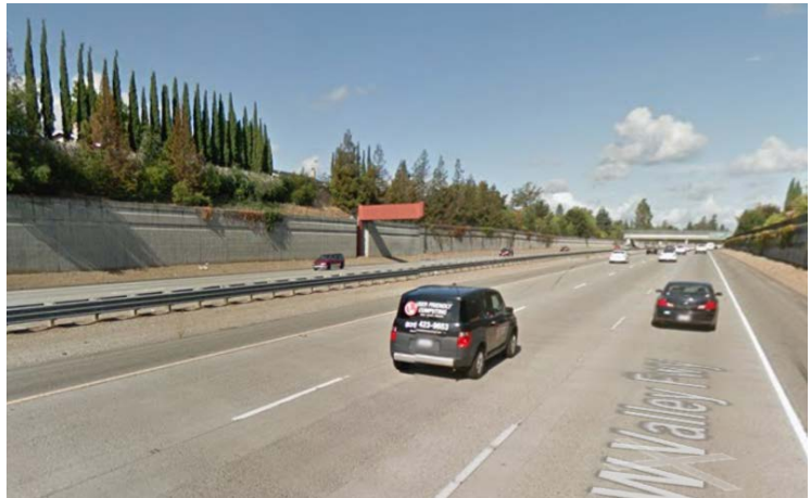
SR 85 below grade, near Cox Ave, Facing North (Source: Google Images)
