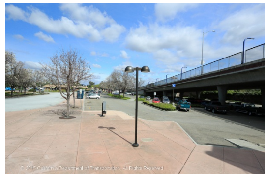
VTA Light Rail Snell Station Park-and-Ride Lot near SR 85
