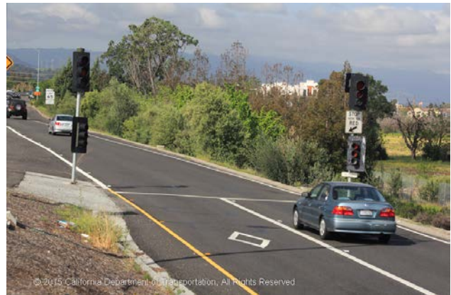
Great Oaks Blvd onramp with carpool lane and ramp metering
