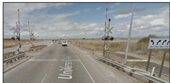
SR 109, facing SR 84/Bayfront Expressway
