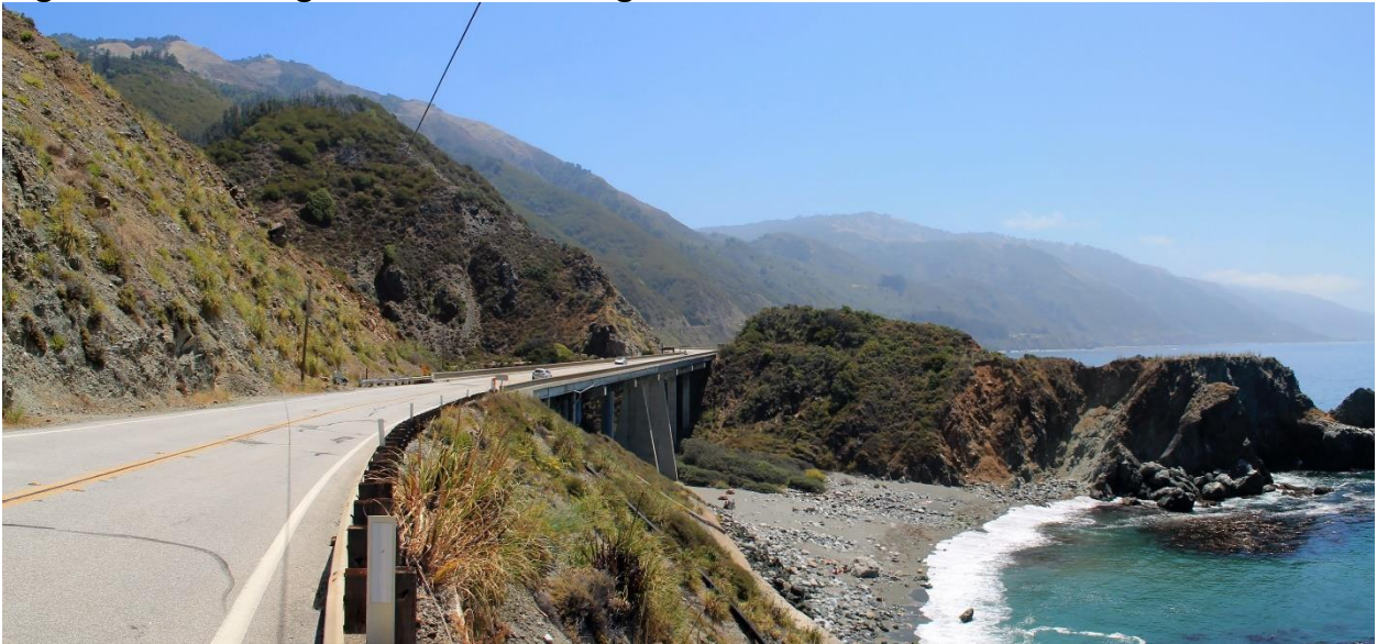
Figure 12 Existing Condition Looking Southbound
