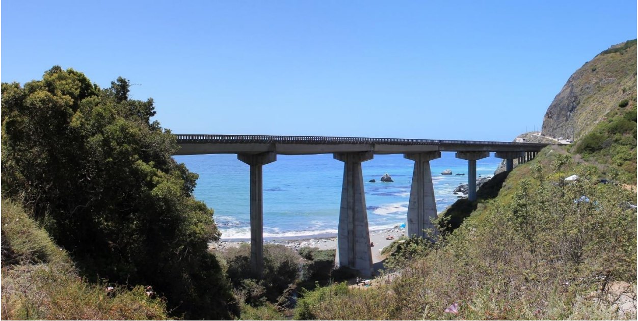
Figure 18 Existing Condition From Entrance Road
