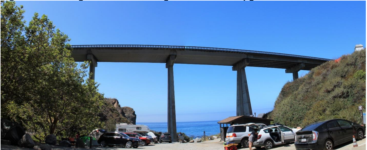
Figure 21 Existing Condition Looking West From Campground
