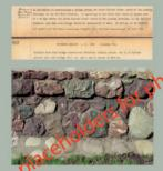
Masonry bridge railings flanked the road surface. Natural rough-hewn stone specially selected for colors of red, blue, and green. topped a unique curved curb embedded with rounded river cobbles
