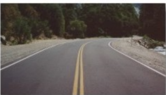
Route 140 after emergency contract repairs (1997 photo) Caltrans partners with contractors to perform emergency repairs when washouts, landslides, slipouts, earthquakes or other emergencies occur.
