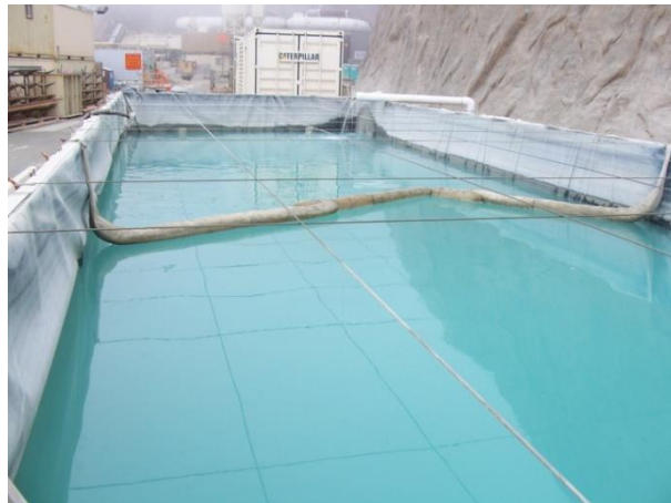
Figure C-2. Sedimentation Tank
