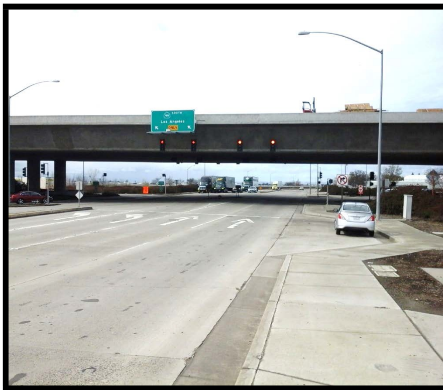
Photo 7: Maintenance Vehicle Pullout Example. SR-99 and Arch Rd.
