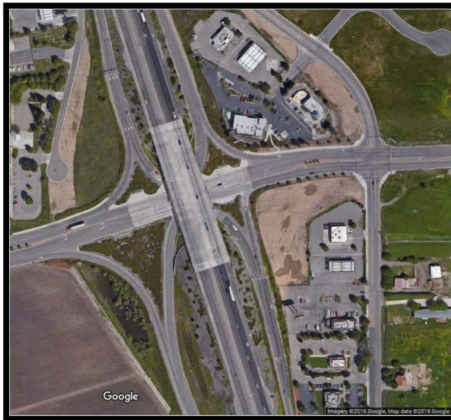
Photo 1: SPI Example. SR-99 and Arch Rd.
