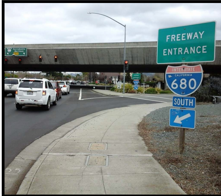
Photo 3: Shoulder and Sidewalk Example. I-680 and Monument Blvd.
