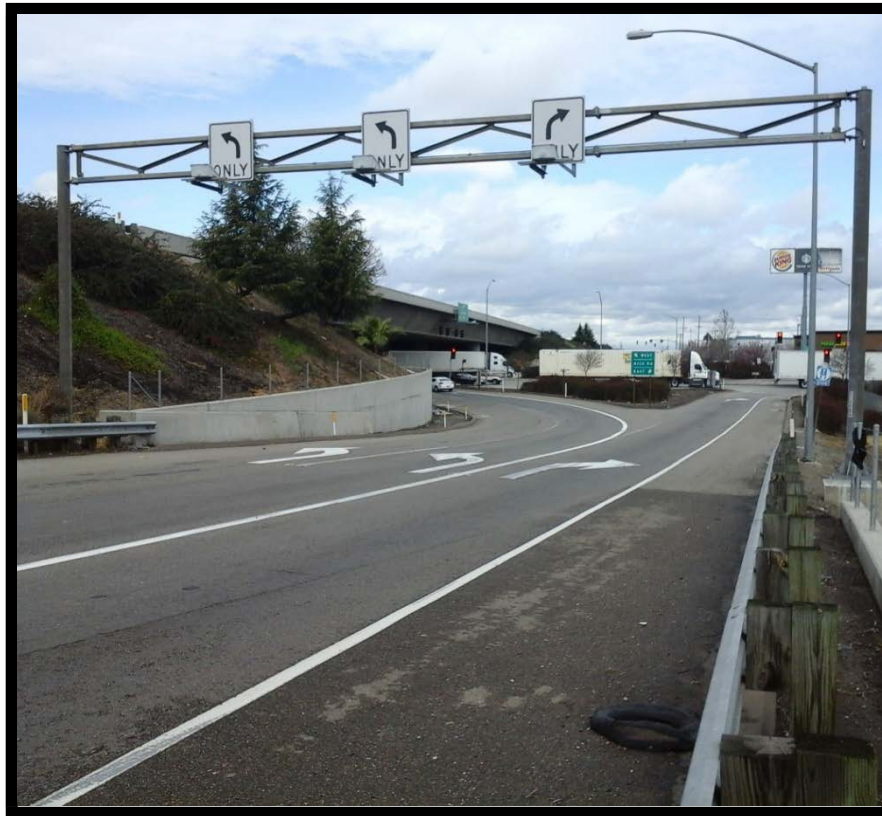
Photo 2: Left-Turn Exit Ramp Example. SR-99 and Arch Rd.
