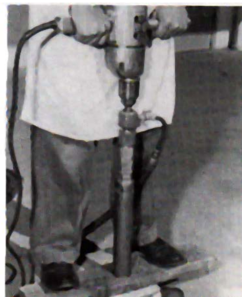
Figure 2: Cutting "Islands" for Testing Overlays
