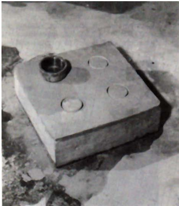
Figure 5: Pipe Bobbin in Place
