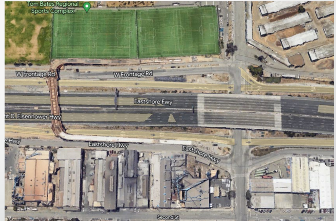
POC Falsework (mid-2022)
