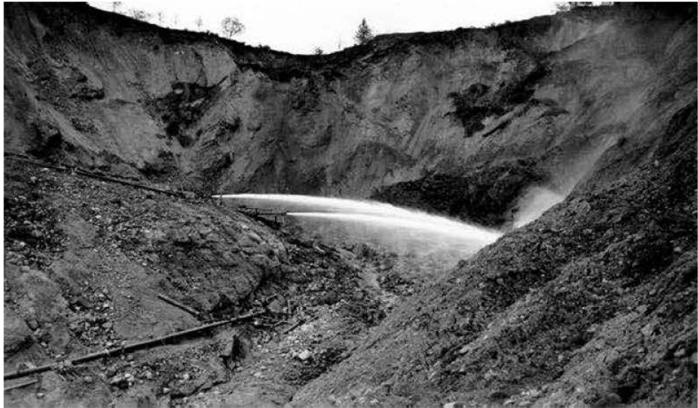
(Monitors in use at La Grange Mine, near Weaverville, California, circa 1940)
