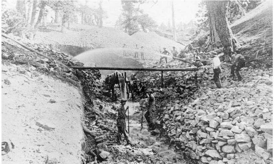
(Monitors in use at Hocumac Hydraulic Mine, circa 1896. Previously published CG, V39, no. 8, p 181)
