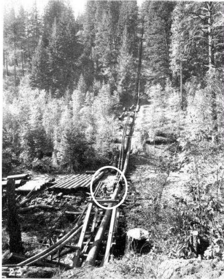
(This photo was taken around 1895 of the La Grange Hydraulic Gold Mining Company's inverted siphon across East Weaver Creek. The Baron and Baroness de La Grange are standing on the left side of the pipeline. Photo on file at Trinity County Historical Society).
