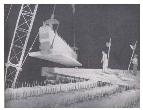
Figure 13: Placing inverted tee beam prestressed girder, San Bernardino-Santa Ana Freeway Interchange, 1955.
