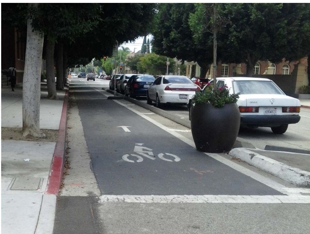
Photo 3: Separated Bikeway with parking curbs and planter in Long Beach
