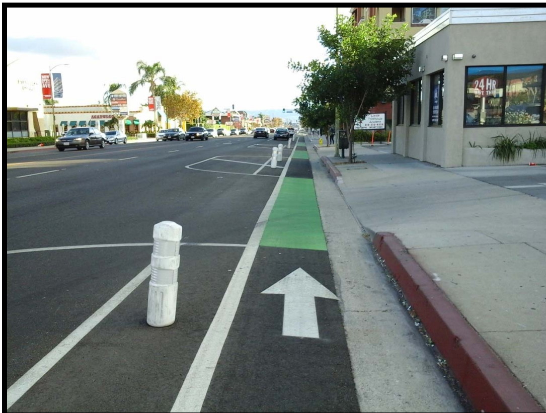
Photo 5: Separated Bikeway with green pavement at driveways in Los Angeles
