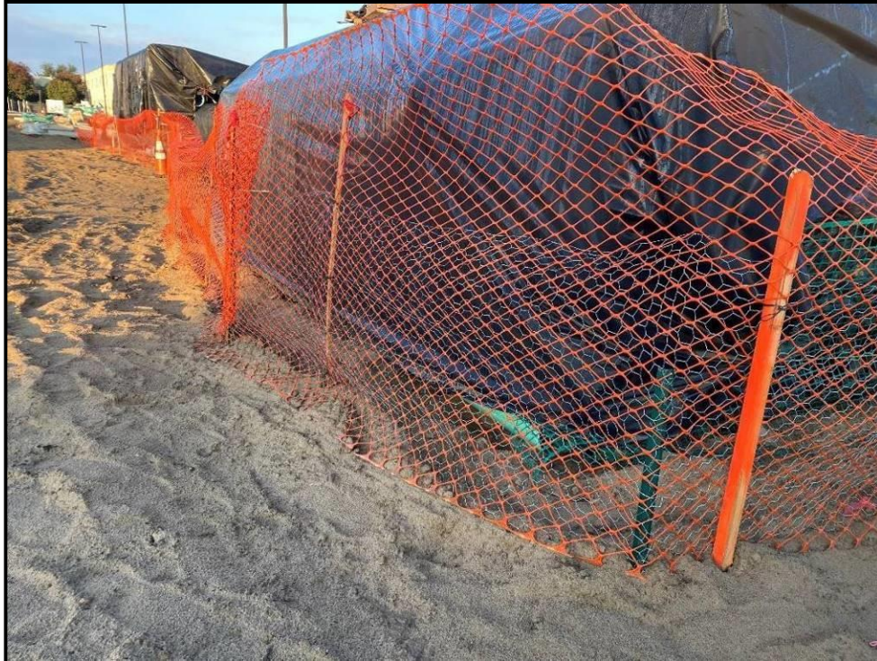
Figure 22. Plastic fencing around construction materials on the Mercy Southwest Hospital study site, Bakersfield, CA, January 2024. Note the layer of metal fencing inside the plastic fence. (Photo by E. Noel)
