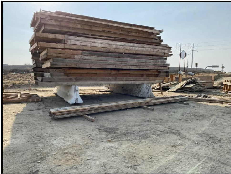
Figure 28. Construction materials placed up on K-rails on the Centennial Corridor study site in Bakersfield, CA, May 2023. (Photo by E. Noel)
