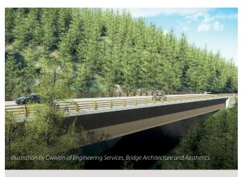
The new Pfeiffer Canyon Bridge in Big Sur, as shown in this depiction, is being rebuilt with steel girders that will span 310 feet across the canyon without need for support towers, eliminating the fear of damage from a landslide such as the one that crippled the bridge in February.
