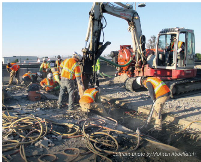
Work crews perform a bridge joint replacement as part of the SR 4 "Big Fix" that made various improvements to the trade corridor.
