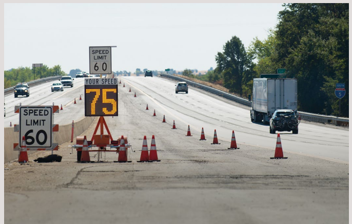
Vehicle Speed Feedback Signs such as this one on I-5 are stationed at work zones to remind motorists how fast they are driving.
