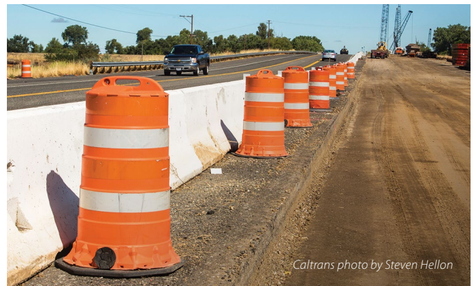
Drums are larger and more visible than traffic cones and not knocked over as often, offering more protection at a construction job site.
