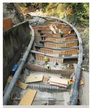
Construction crews complete framing on the fish passage structure built on Cedar Creek, outside the town of Leggett on the North Coast.
