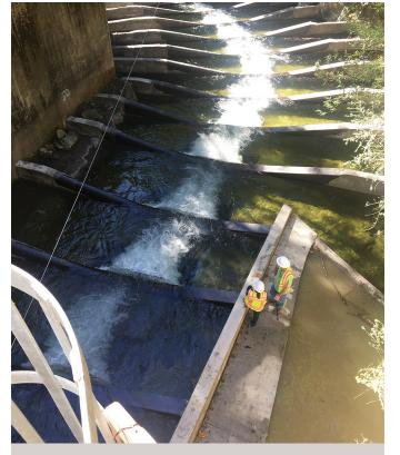
The finished passageway consists of a series of 13 gradually descending steps, replacing a previous weir structure that had deteriorated.
