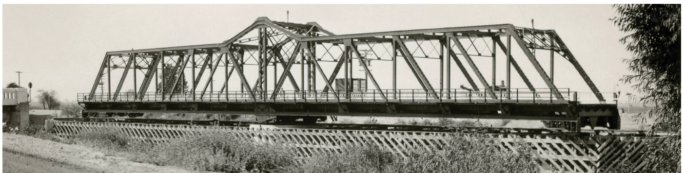
The Garwood Ferry Bridge opened in 1934 across the San Joaquin River in Stockton, connecting that city and the Central Valley to Contra Costa County and the East Bay via State Route 4. Built as a swing bridge that rotated on a central pier, the Garwood Bridge no longer opens for boat traffic.
