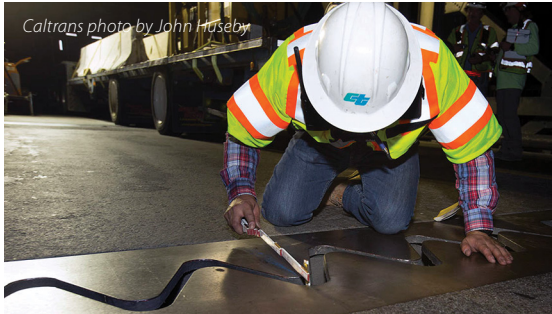
Caltrans' Alfredo Carranza measures joint tolerances on the Rio Vista Bridge during a recent round of repairs.
