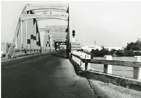
The Rio Vista Bridge, pictured in 1952, would undergo a major rebuild from 1957-60 into its present configuration. The original bridge opened in 1919 no longer exists.
