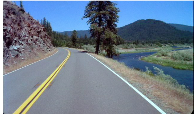
Figure 26: SR 96 is a curvy two-lane highway without shoulders -- run off the road crashes are common.
