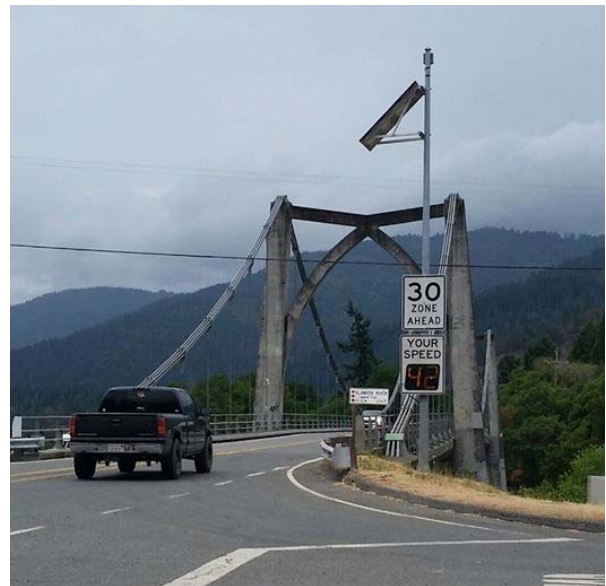
Figure 23: Through a cooperative traffic calming effort of the Karuk Tribe and Caltrans D1, radar speed signs were installed in the community of Orleans, CA
