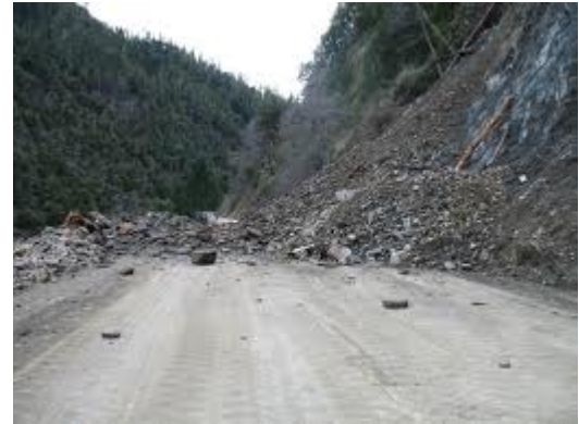
Figure 17: SR 96 near Somes Bar, CA. Landslides and falling debris are a common occurrence.
