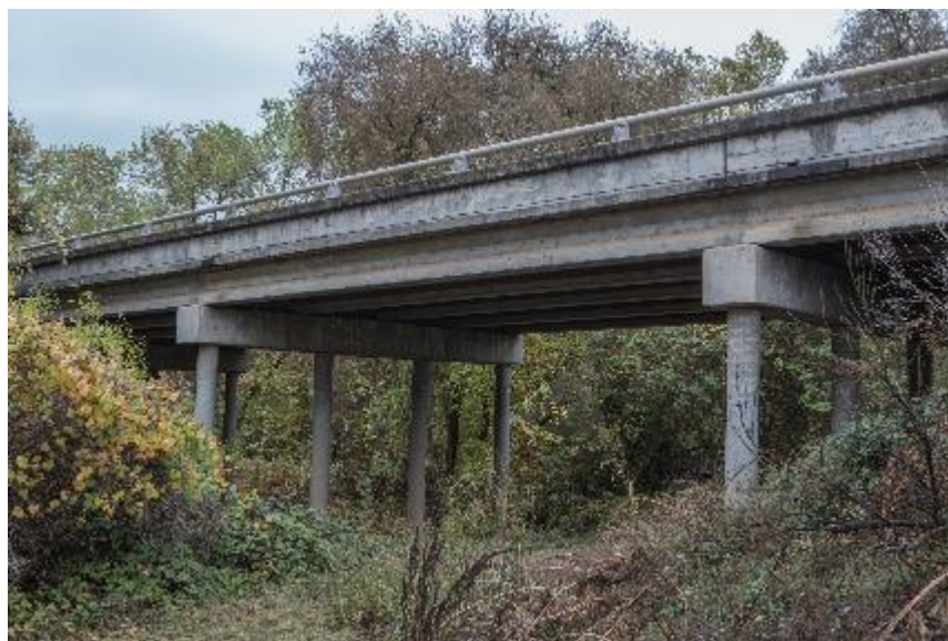
BUTTE CITY BRIDGE, HIGHWAY 162
