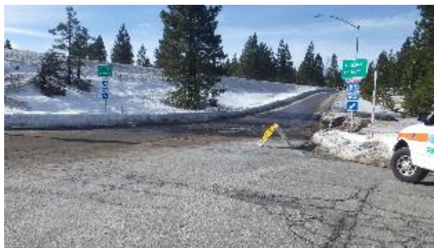
I-80 RAMP REPAIR NEAR NYACK
