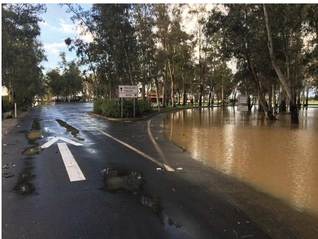
FLOODING AT WILLOW REST AREA
